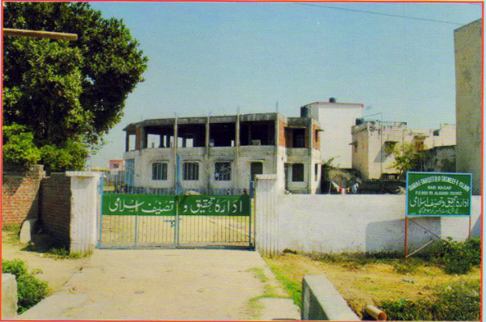
Main gate of Idara
